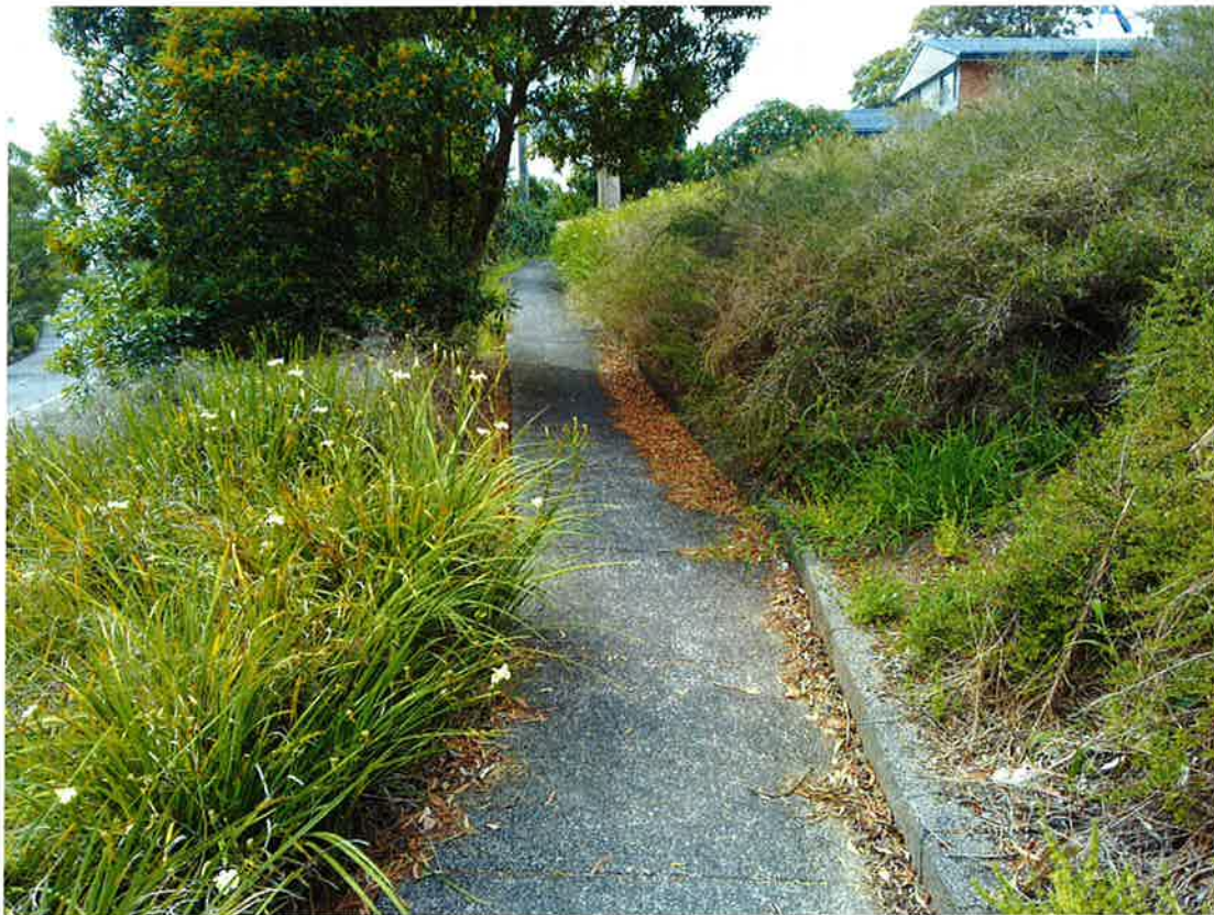
Photograph 5 – Concrete Footpath to Wyong Road
